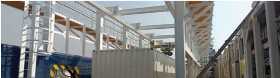
FABRICATE & WELDED SPOOLER FRAME STRUCTURE WITH WALKWAY PLATFORM FOR ROPE STORAGE CONTAINER.
